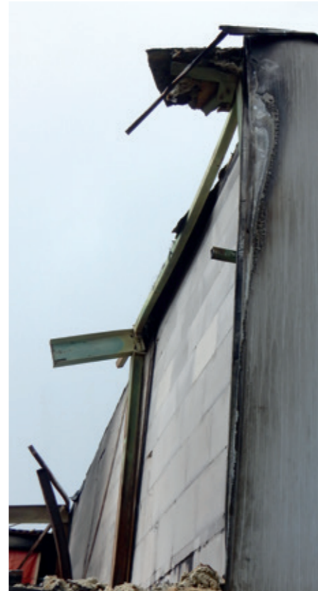
Panel at junction with internal compartment wall.
