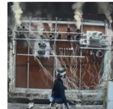
Test for 1 hour penetration seals.
