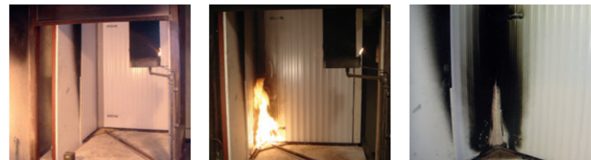
Test set up During test End of test showing minimal panel damage
