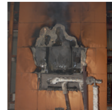
End of test demonstrating damage to ACM rainscreen with Kingspan insulated metal panels remaining intact
