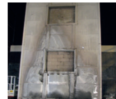
Façade after test demonstrating minimal fire spread attributable to the cladding
